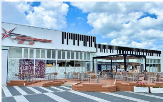
NEOPASA HAMAMATSU SERVICE AREA
